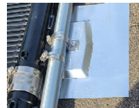
HOT SUN STRAP BRACKET HOT SUN #20 ALL SS GEAR CLAMP 1.375" OD CHAIN LINK FENCE TOP RAIL
