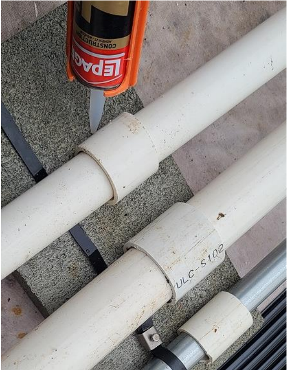
Slip collars glued to ballasts (flat roofs)
