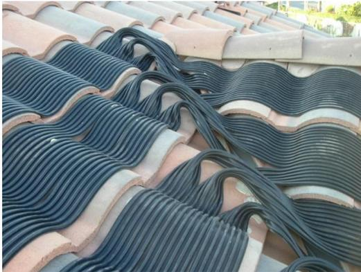
If you strip the 6 tube wide strips into individual tubes you can twist it to go around bends as shown above right. Separating into individual tubes at the end and attaching each tube individually to the header allows you to angle the headers. The headers do not need to be perpendicular to the flow!
