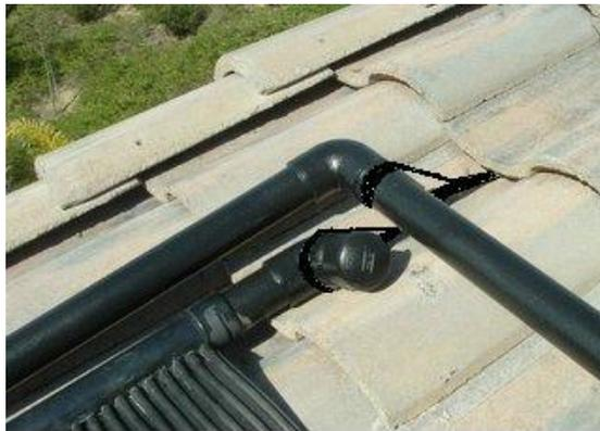
One good way is to slip ppa coated ss strap through a strap bracket as shown above left. Then just slip it between tiles (lift tiles with a screwdriver) . Note we glued the cap to the end of the row of headers via an elbow so we had an easy way to hang it. Another good way is to secure to the wood you will find under the ridge cap as seen below left..
